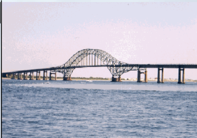
This 1999 photo shows the single-span Robert Moses Causeway bridge crossing Fire Island Inlet. (Photo by Steve Anderson.)
